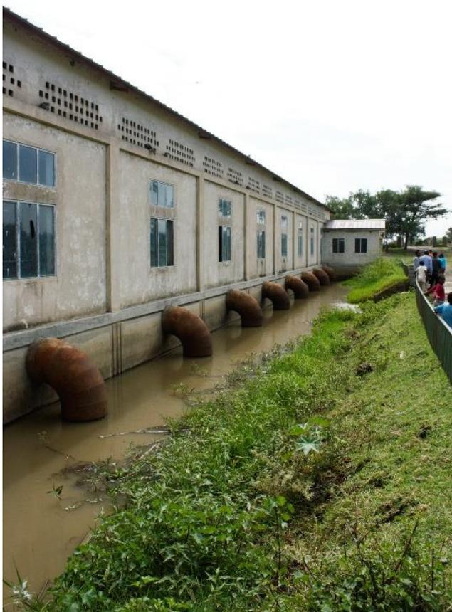
*Figure 21 Poor condition of basin pumps of the pump house*
