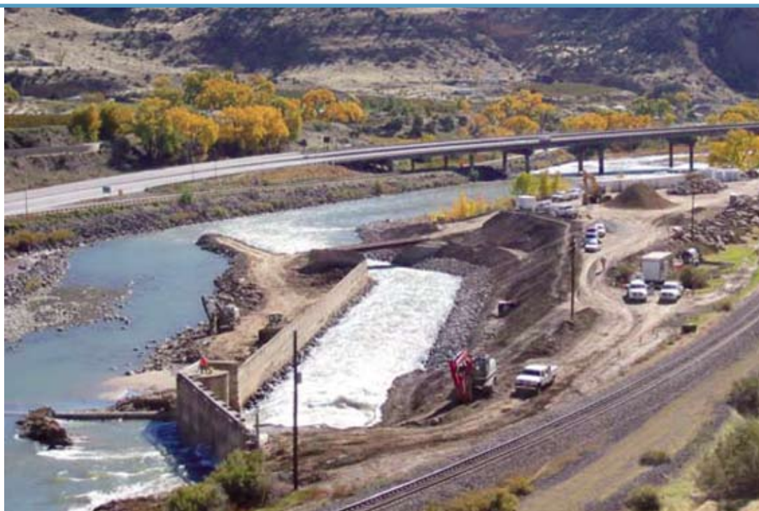
Figure 1. The Price-Stubb Diversion Dam fish passage on the Colorado River near Grand Junction, Colorado, was completed in 2008. Removal of this barrier to fish migration provided endangered fish access to an additional 84 km (52 miles) of critical habitat that had been blocked since 1911.
